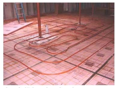
Since the floor has tubing running approximately 2" down throughout the floor, you cannot cut the floor for tension relief.
