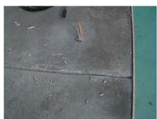
Once the strip is in place, a mixture of the 105 grout and 111 modifier is used to set the strip in place. This is done by pouring the mixture into the channel around the strip and troweling smooth. Once this is dry, you can skim the deck and install the CTI System as usual.
